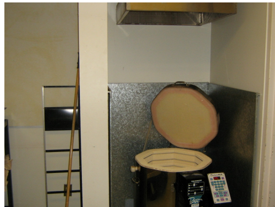
Kiln has an existing exhaust hood but inadequate exhaust.
