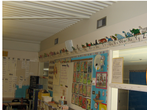
Classroom supply air grilles. The return air is typically behind the valance (has the alphabet on it in this photo).
