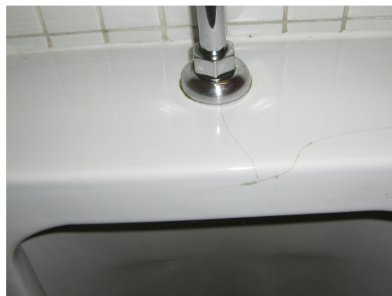
Crack at top of urinal.
