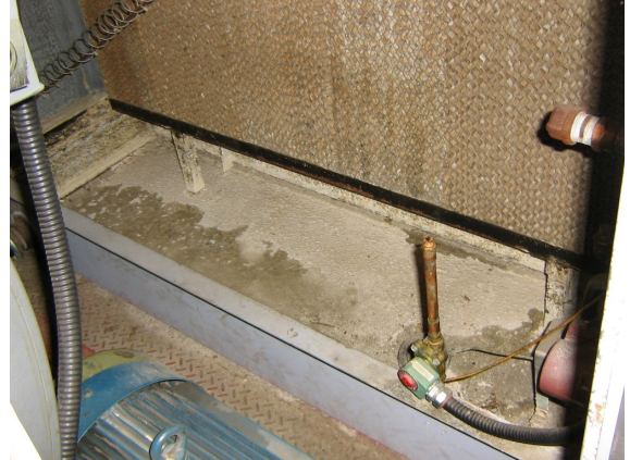
Abandoned humidification media in AS-2.
