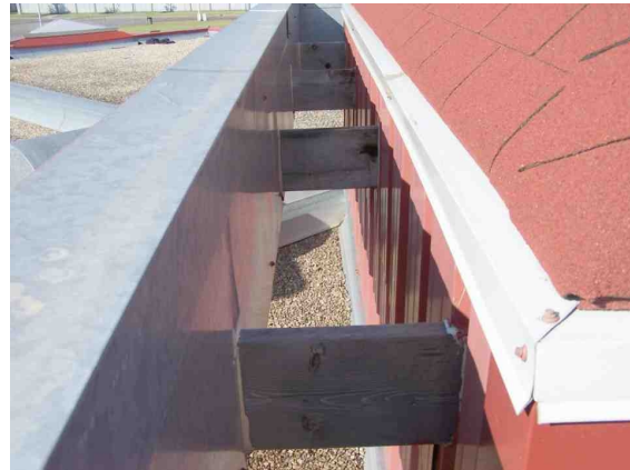
Exposed wood left to weather; left unprotected future repairs costs will be greater.
