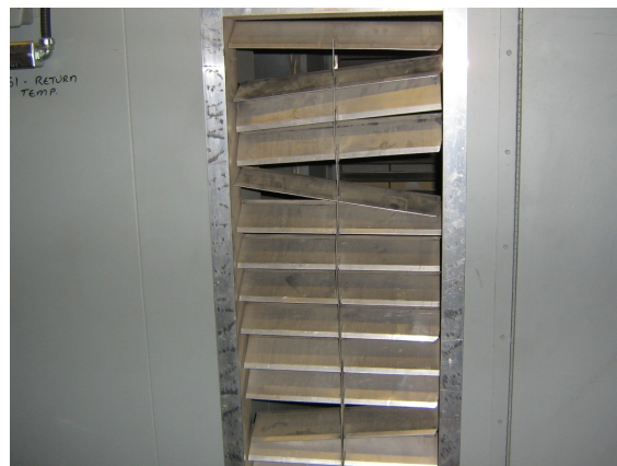
Damaged damper.
