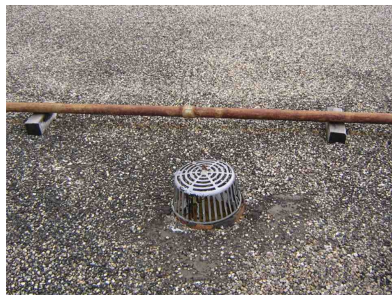
Gas line on roof is rusted.
