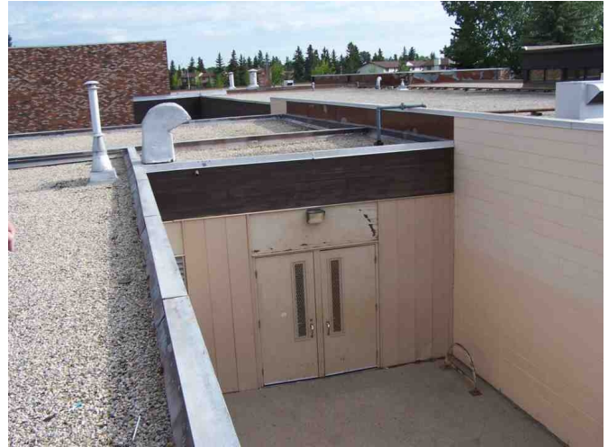
Painted concrete block (firewall) at end wall of permanent construction.
