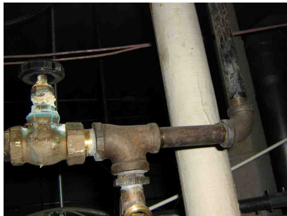
Valve at the coil evidence of leaks.
