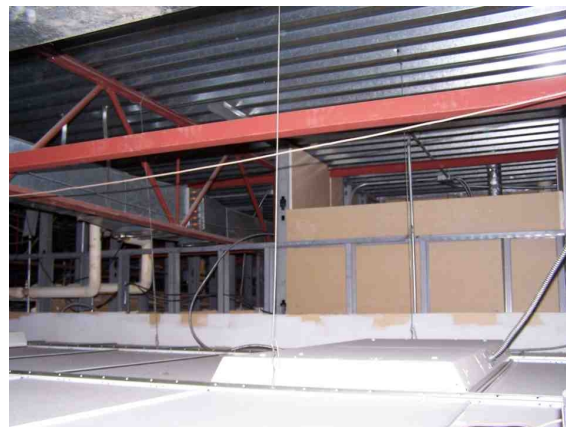
Fire separations are incomplete.
