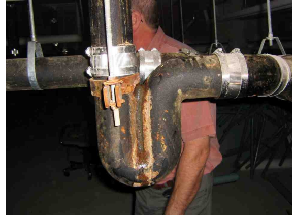
Trap leaking in crawl space.
