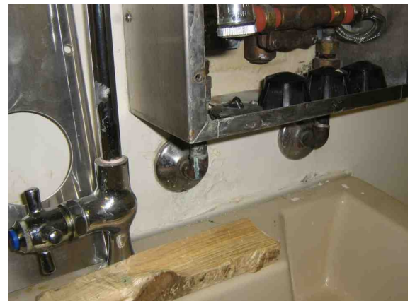
Mixing valve leaking.
