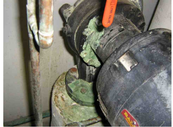
Evidence of pump leaking.
