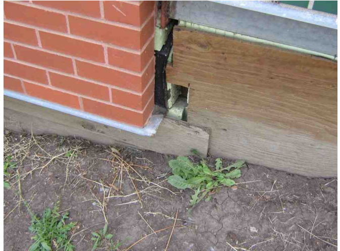
Unfinished wall/ insulation protection.
