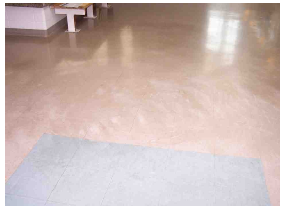
Flooring wear surface is worn off.
