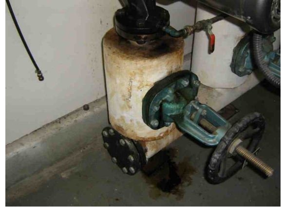
Leaking valve has damaged the insulation around it.
