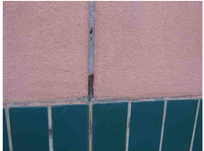
Sealant failure/separated.
