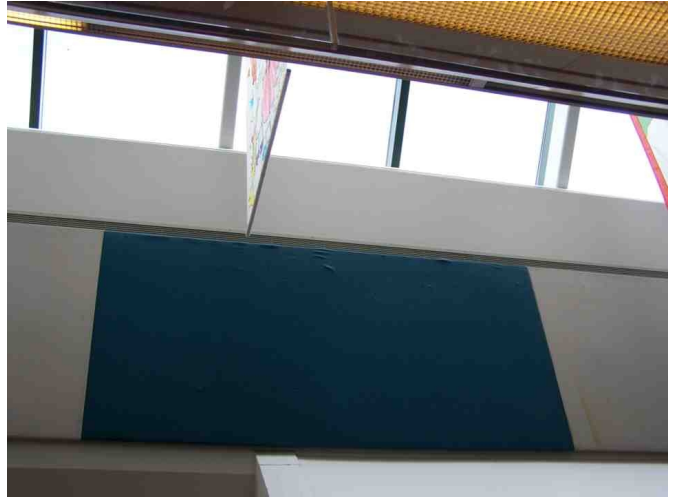
Water stained acoustic panels.
