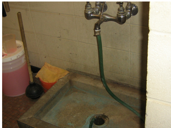
Existing floor mounted service sink.
