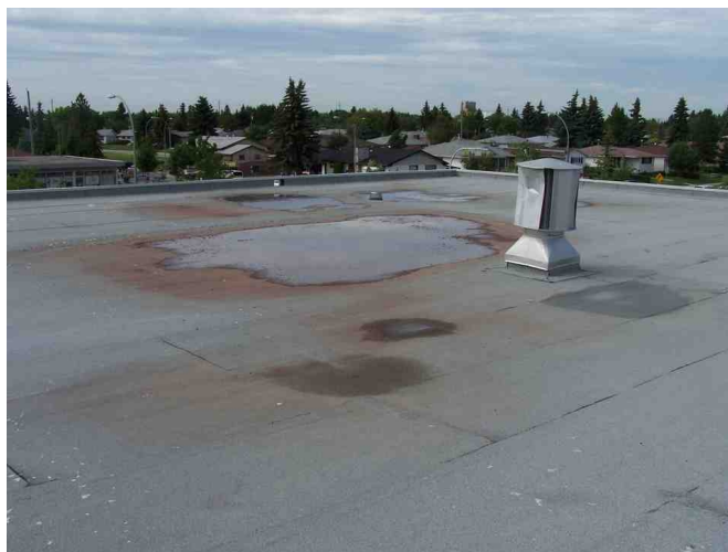
SBS Roof on Upper Gym Roof - 1958 Section.
