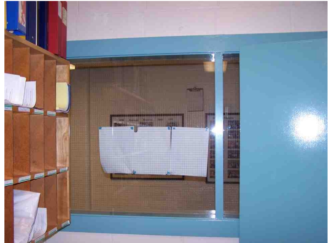
GWG glass in workroom in 1958 Section.
