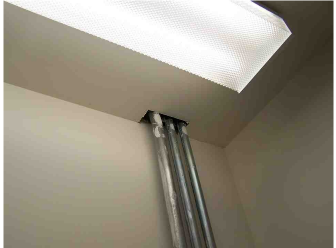
Unsealed pipe penetrations - typical.
