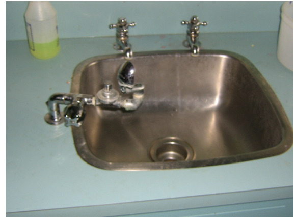
Existing classroom sink with separate supplies.
