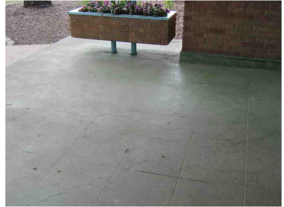
Walkways have cracks
