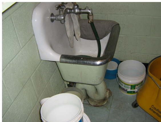
Existing service sink require lifting buckets to empty them.
