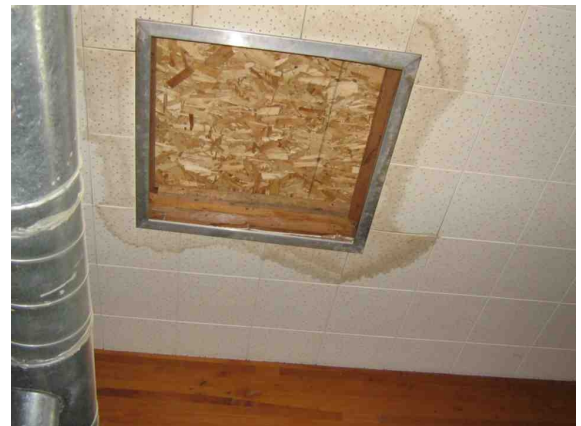
Roof opening that has been boarded over.
