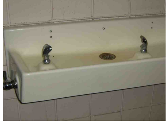
Typical existing drinking fountain. Notice the screws in the back holding it to the wall.
