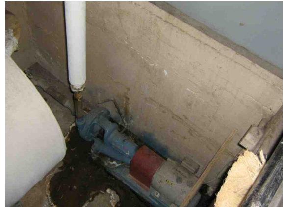
Domestic water circulation pump.
