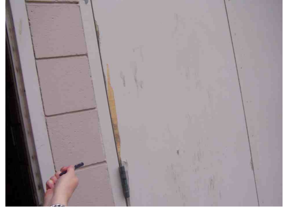
Wood door- delaminating.
