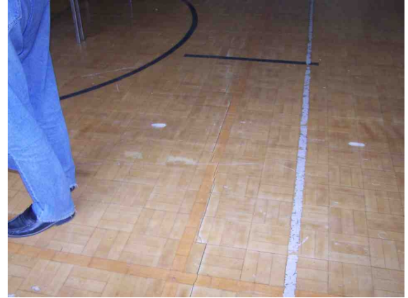
Gymnastics - flooring is crack, and various surface damaged areas.
