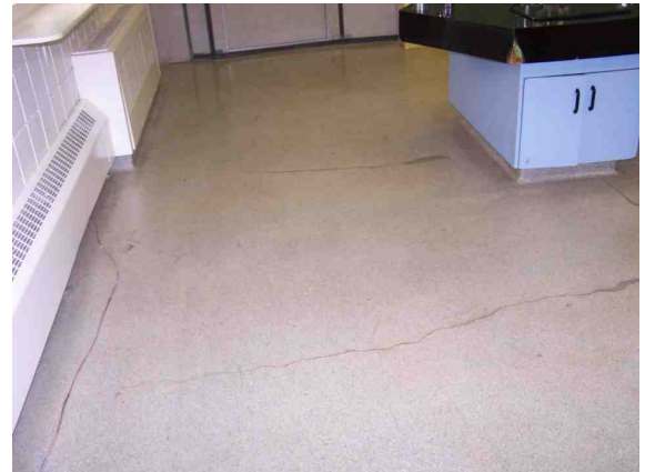
Cracks in epoxy flooring.
