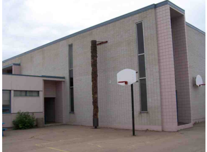
Concrete block with brick veneer - 1967 Section.
