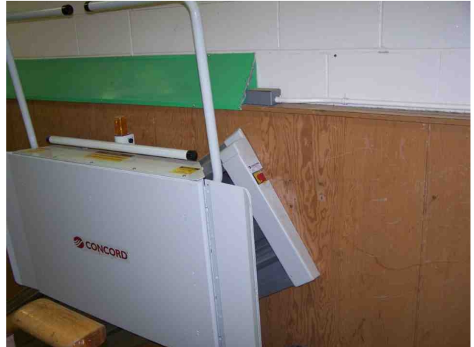
Stair lift at stair to access the main gymnasium.
