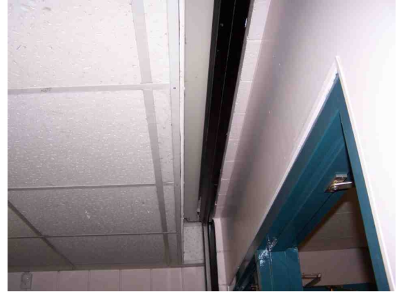
2 rolling shutters- one at each side of wall; door swings will not permit shutters to close.
