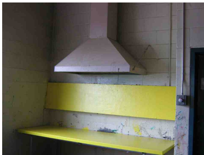
Exhaust paint fume hood.
