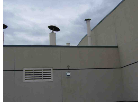
Chimney cap is damaged.
