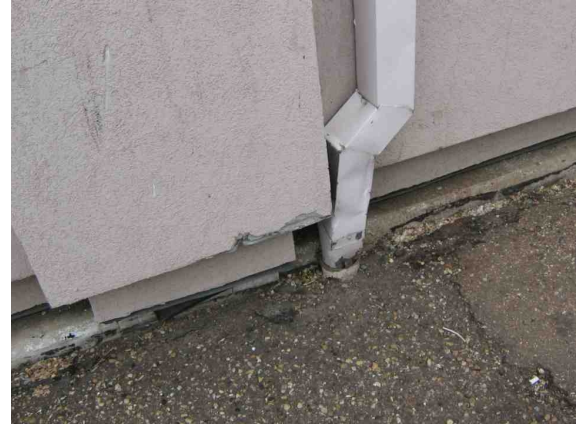
Damaged rain water leader.
