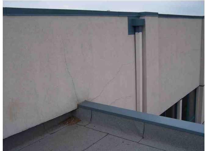
Stucco cracks
