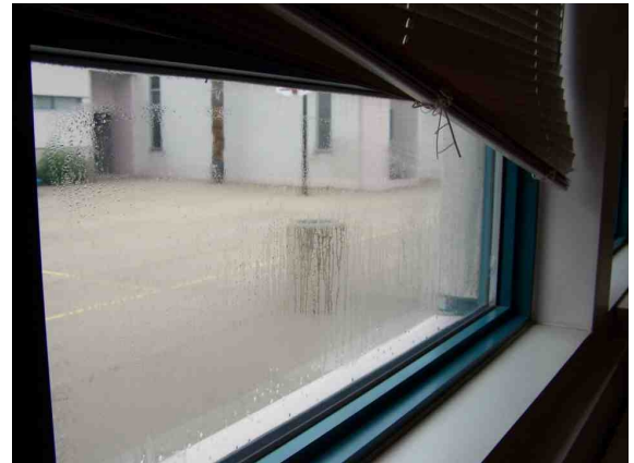
Moisture build-up between glass panes.
