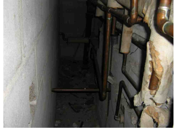
Damaged insulation.
