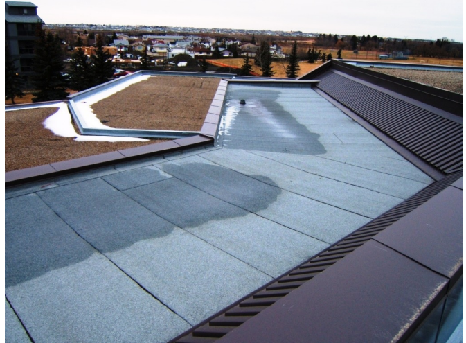
SBS membrane roofing.
