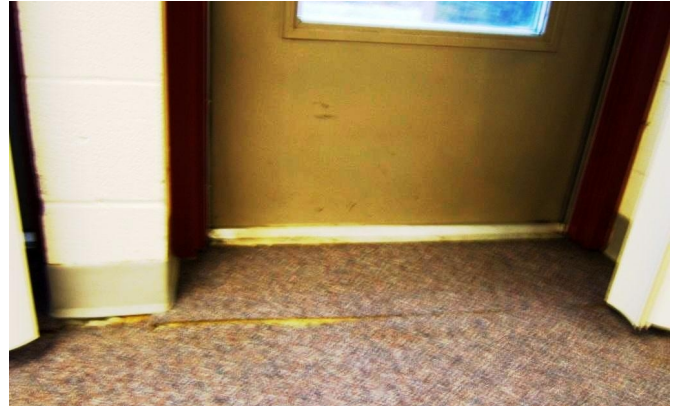
Floor crack at exterior access to music room.
