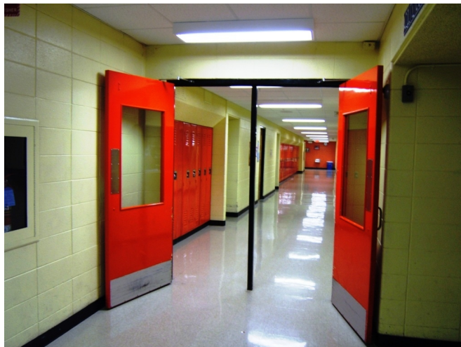
Fire doors complete with magnetic door holders and glazing units.
