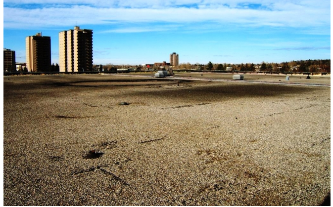
View of built-up roof assembly.
