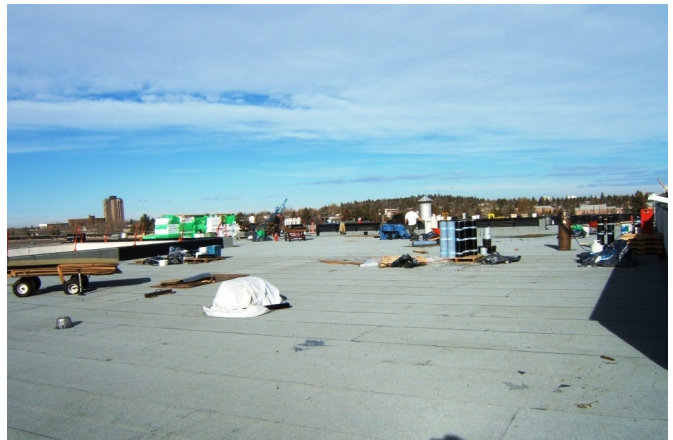
View of SBS assembly being installed.
