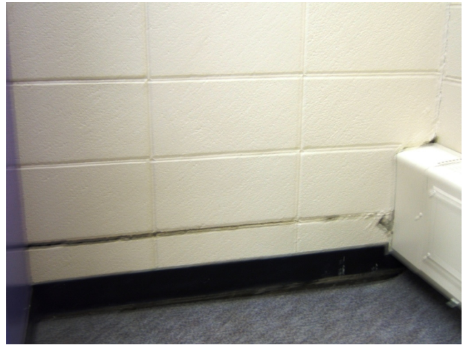
Settlement crack in southwest corner of Room 28 on main floor.
