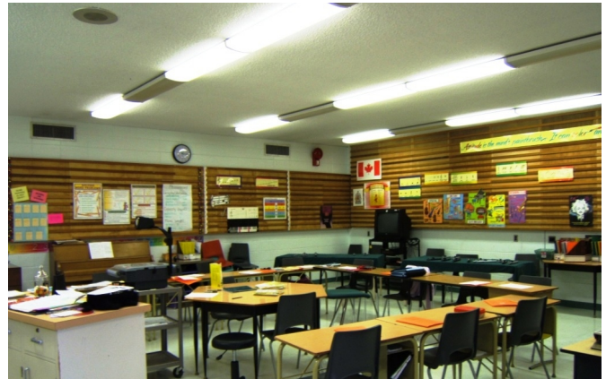
Stained wood acoustical paneling.
