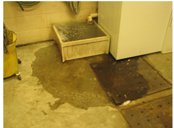
Water overflowing from mop sink as washer discharges water into broken sink. Location: Custodial.
