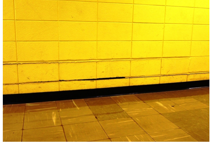
Settlement crack in Corridor C-5 on second floor between Auto Repair and Metal Working Shop.
