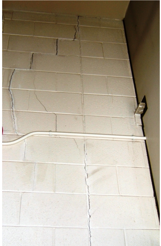
Wall crack in main floor storage space.
