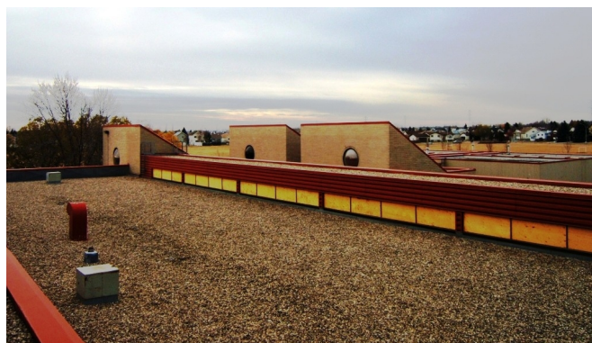
Partial view of roof with boarded up clearstory windows.
