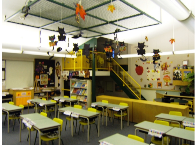
Painted metal balustrades and handrail to classroom study space.
