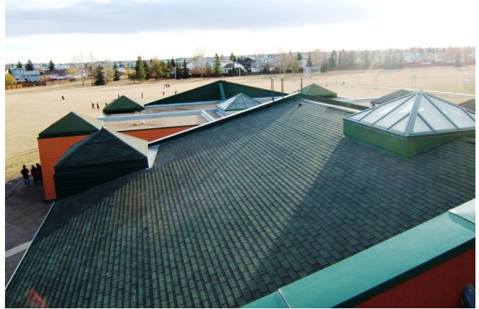
Partial view of asphalt shingled roof.
