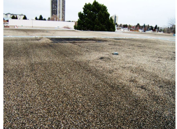
Partial view of roof with visible roof patch, area divisions and metal flashing.
