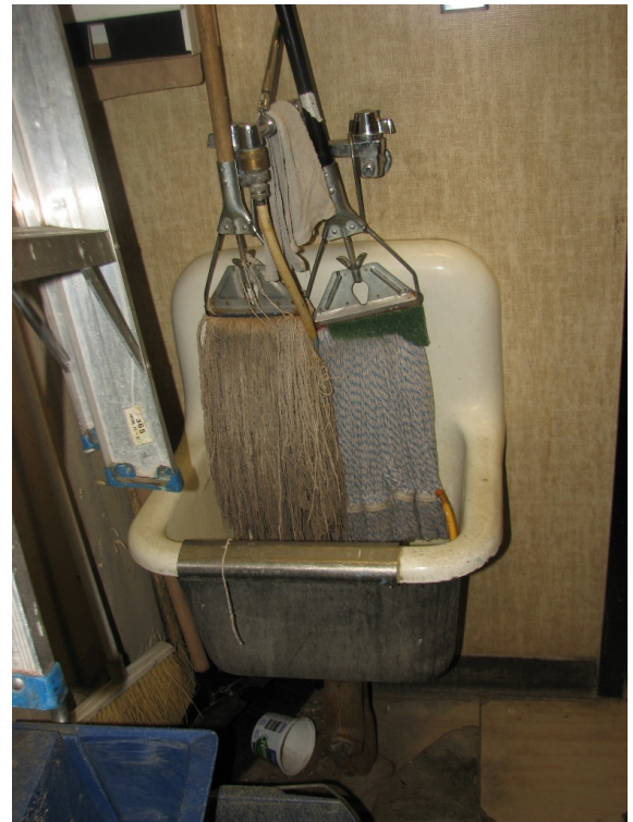
Wall hung mop sink in need of failure replacement.
