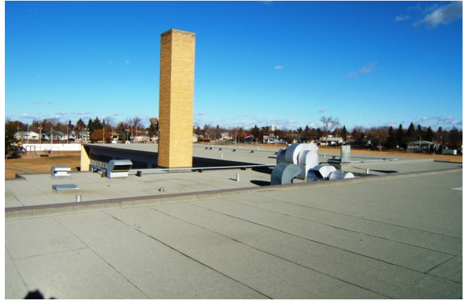
View of roofing elements.
