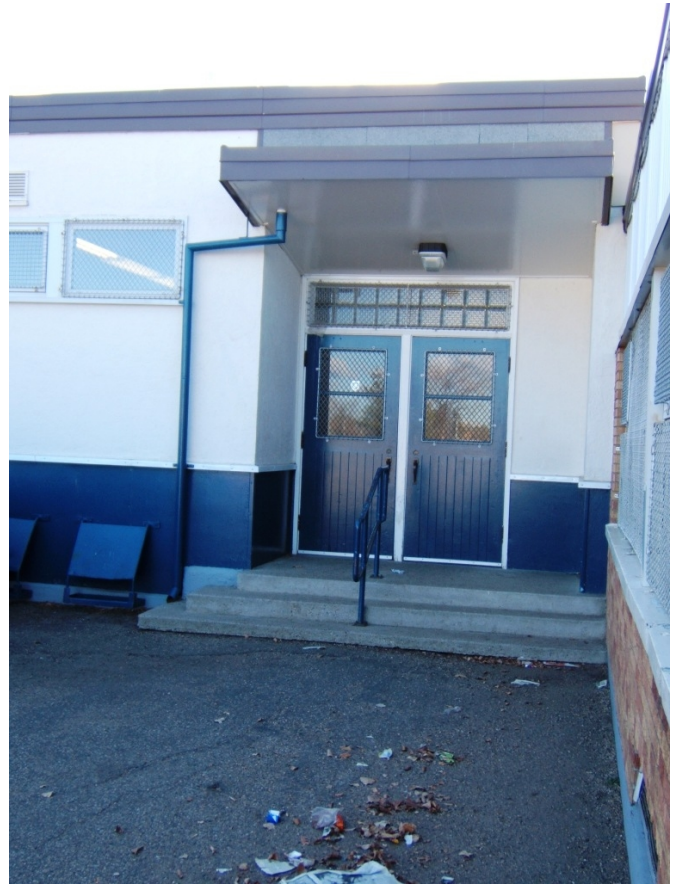
Concrete stair to vestibule.
