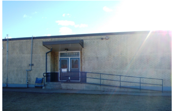
Concrete ramp and stairs.
