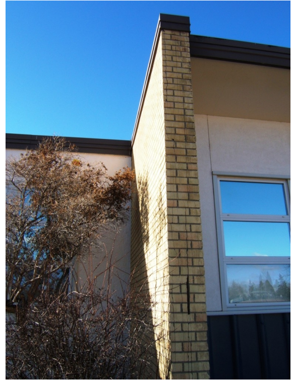
Typical brick clad wing wall.
