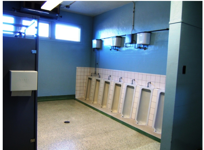
Boys wash room finishes.
