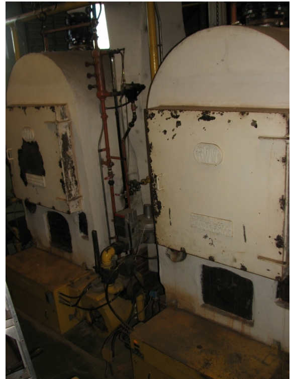
Boilers show signs of corrosion.
