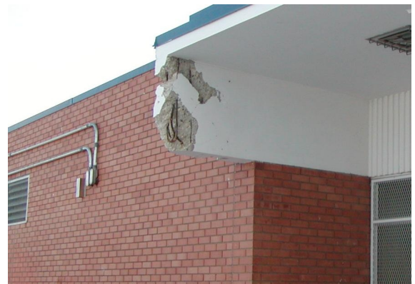
Cast in place concrete overhang at north west entrance.
