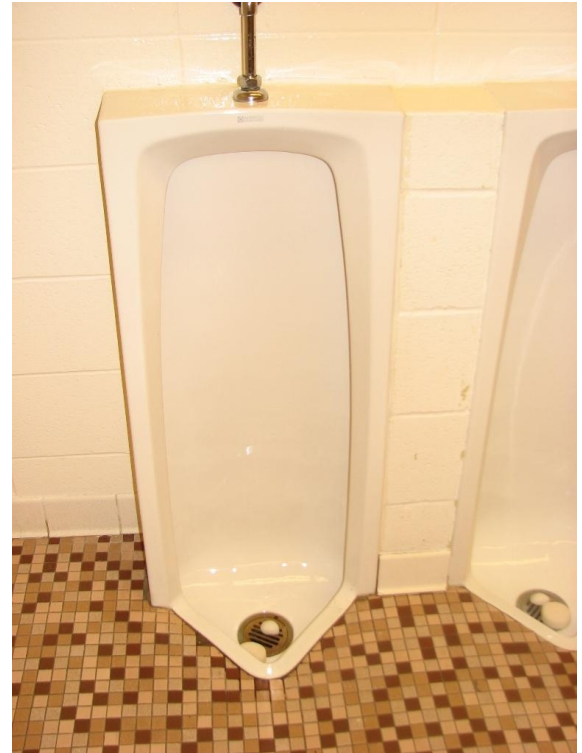
Typical American Standard, tank type urinals.
