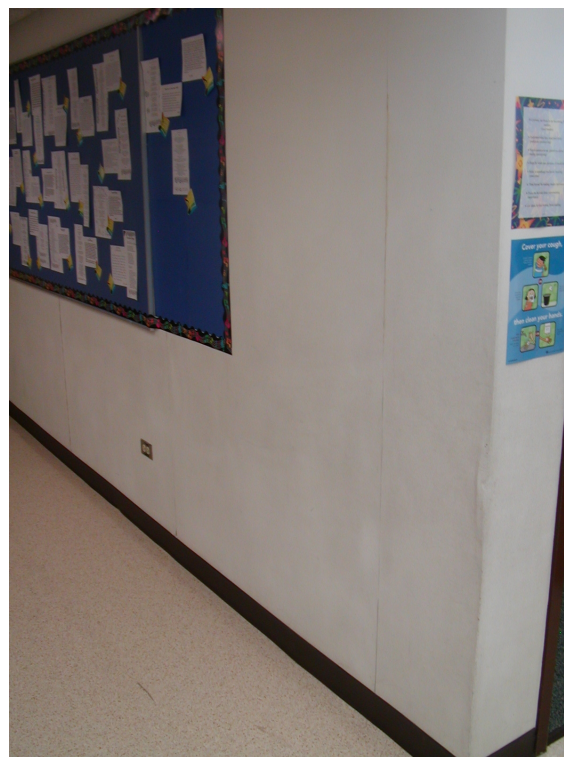
Vinyl wall coverings in corridor c10.
