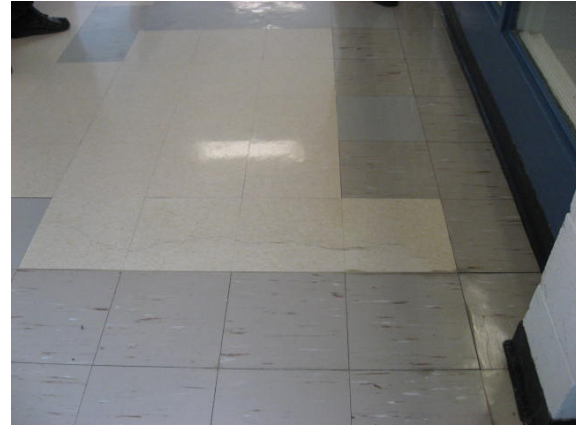
Vinyl floor tile on the second floor corridors
