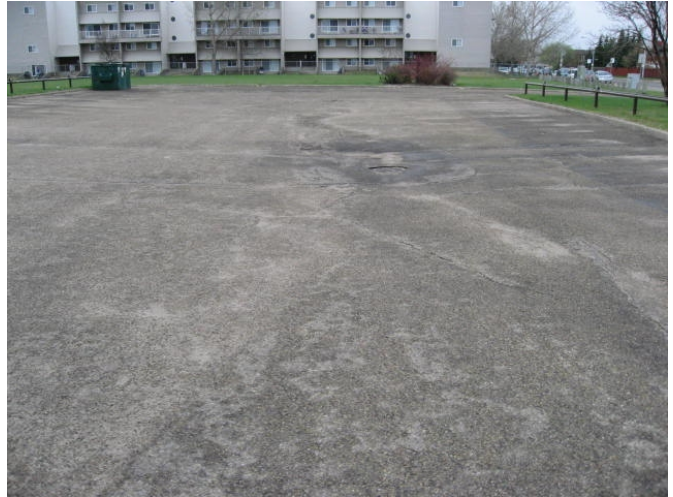
Asphalt paved parking area with extensive cracks and settlement.
