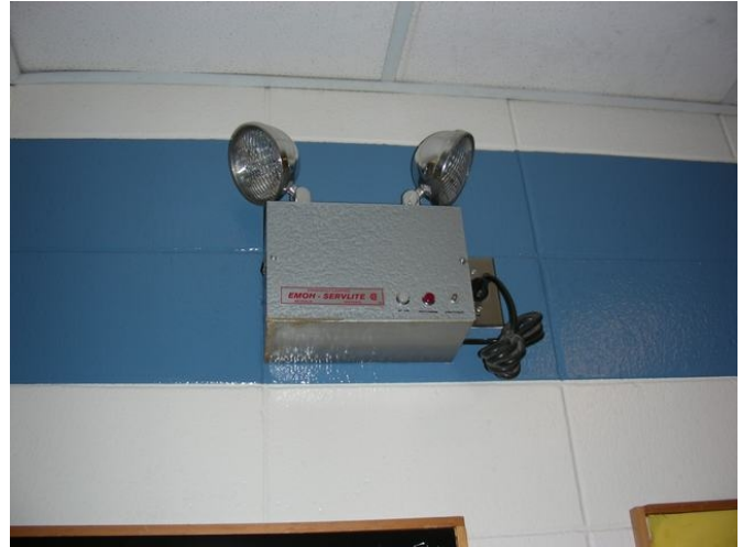
Aged emergency lighting battery pack.
