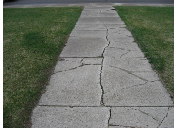
Cracked concrete walkways at the north-west end of the site.
