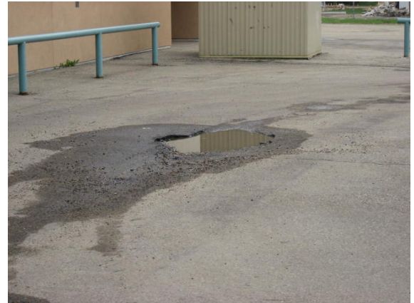
Sinkhole in parking area.
