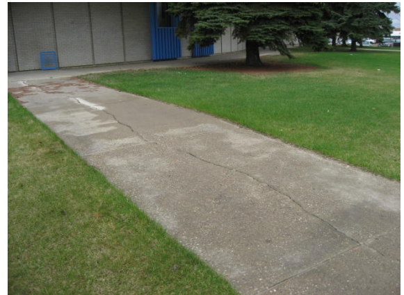
Cracked poured concrete walkway.
