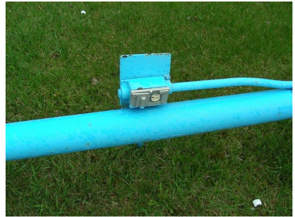
Damaged coverplate on car plug-in.
