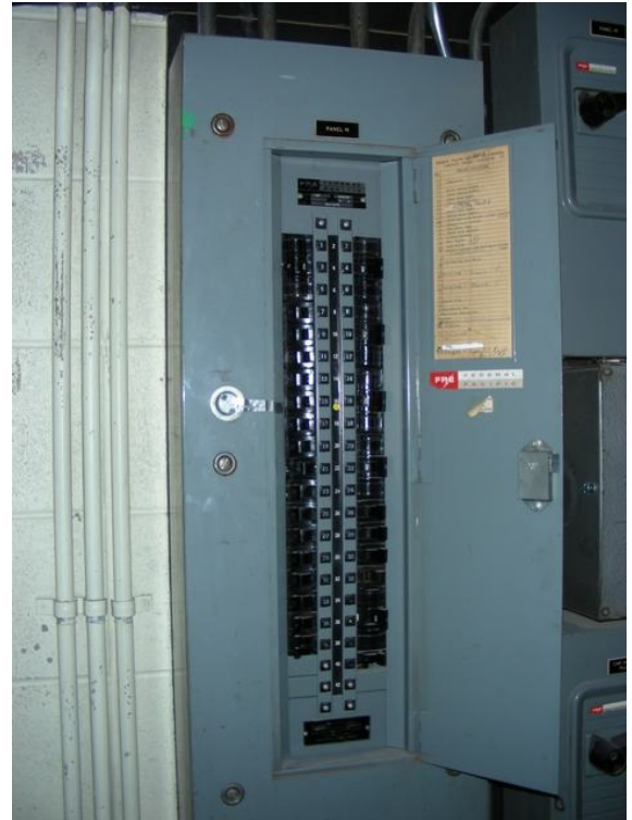
Aged branch circuit panelboard.
