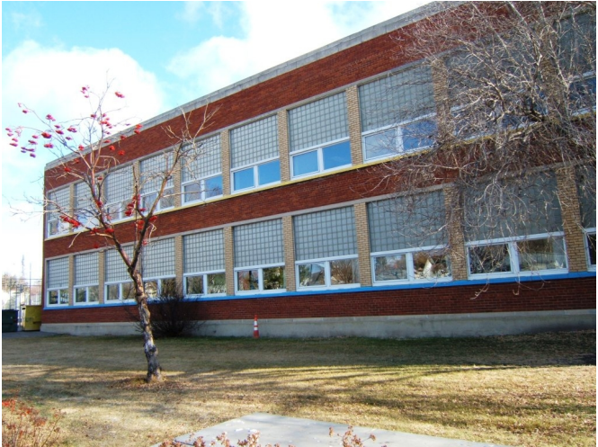
View of glass block over window units 1952 Section.
