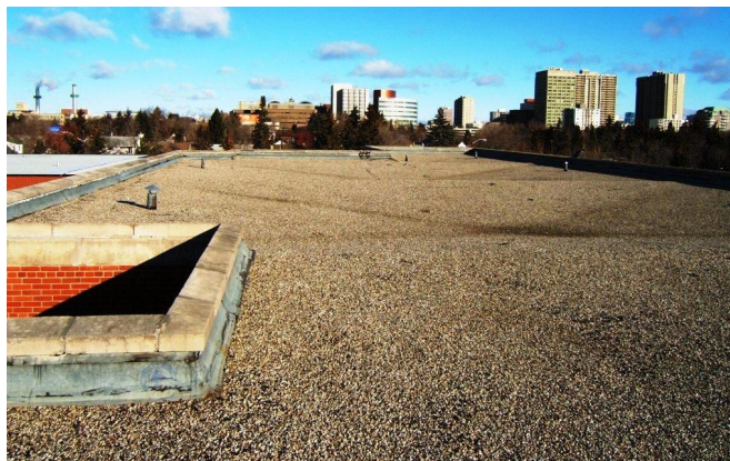
View of asphalt built-up roofing - 1952 and 1953 Sections.
