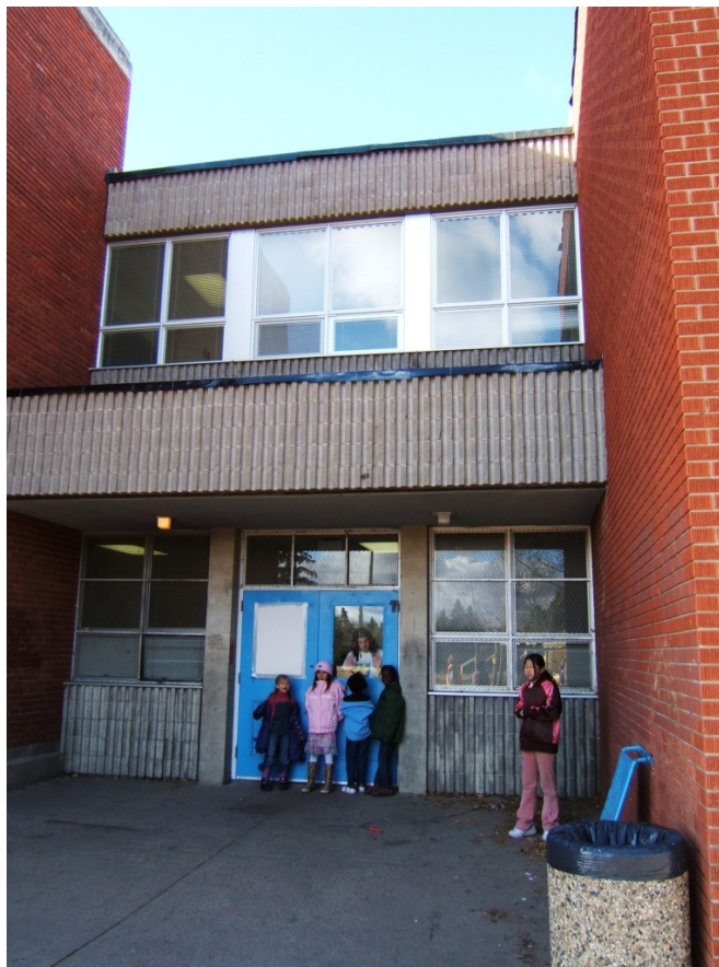
Precast elements at east entrance to 1973 addition.
