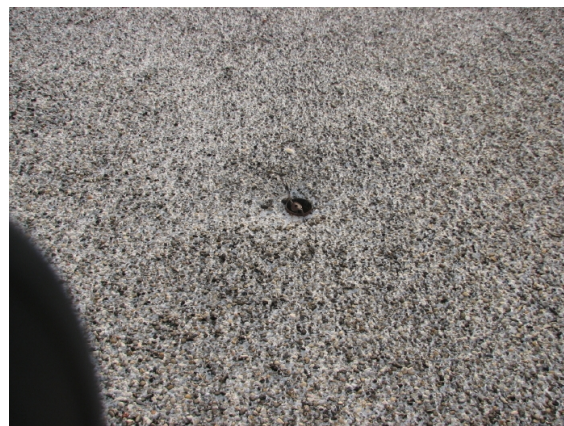
Typical condition of Roof Drains serving the school.
