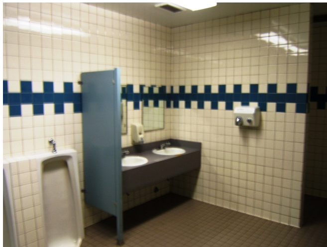
Typical upgraded washroom.
