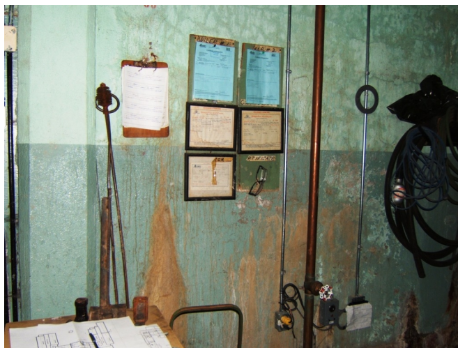
Exterior mechanical room wall.
