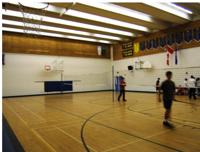
Stained wood wall panels in north gymnasium of 1973 Section.
