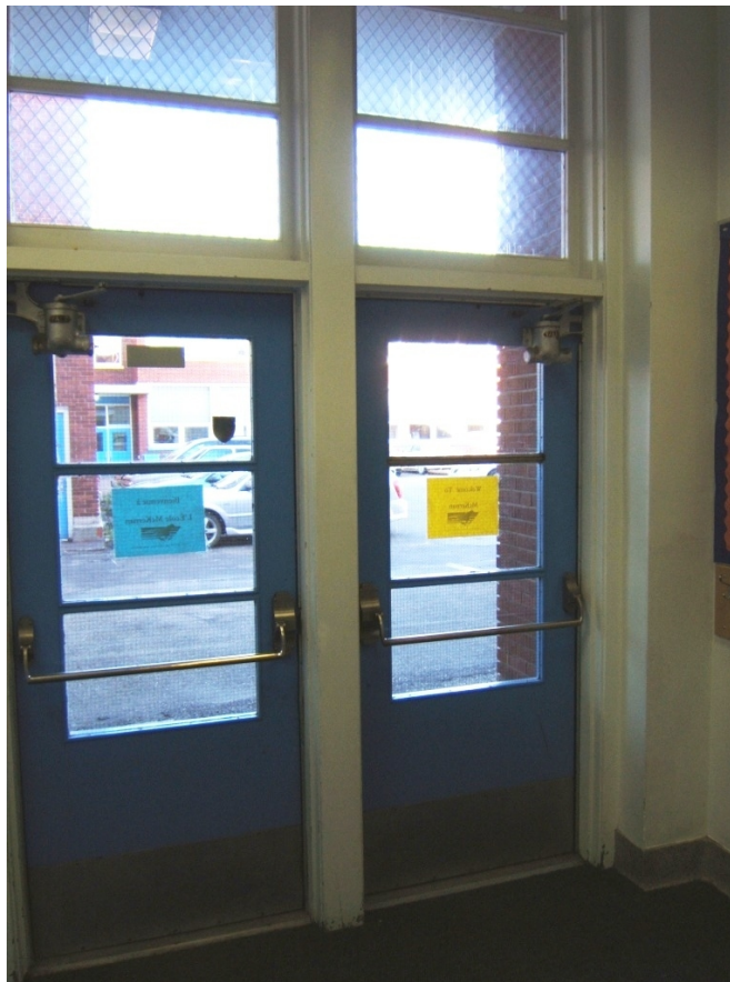
Typical exterior entrance doors all sections.
