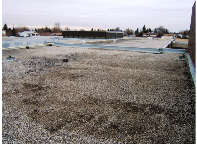
Partial view of built-up roofing.
