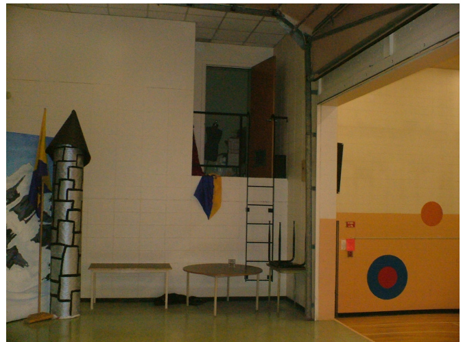
Steel railing for mezzanine above gym storage room at stage. A wall-mounted steel ladder from stage to mezzanine.
