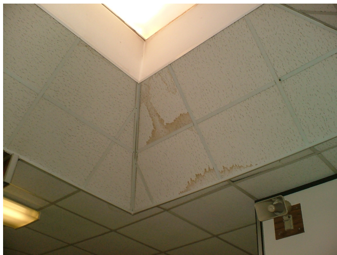
Water stains on ceiling tiles below the skylight.
