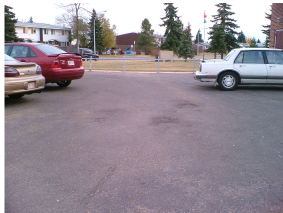
Pot holes and cracks in parking lot.
