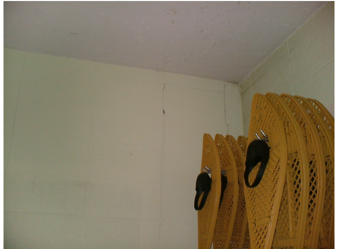
Cracks on the concrete block wall in the gym storage room.
