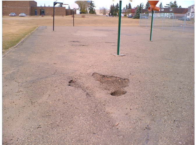
Asphalt pavement with cracks and pot holes.
