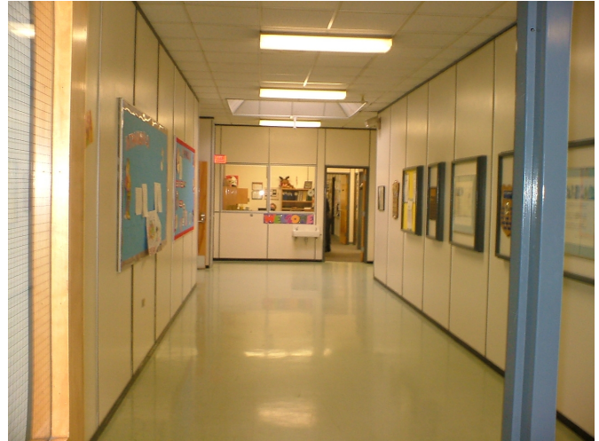
Gypsum board with vinyl wall covering on metal stud frame partitions.
