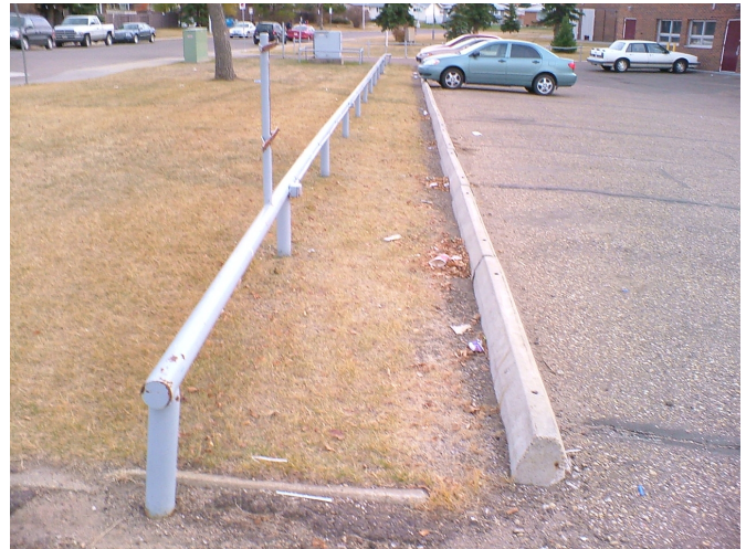
Precast concrete bumpers for the parking stalls on the east side of the parking lot facing the lawn.
