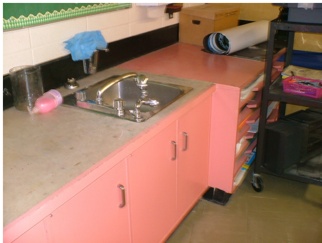
Painted plywood casework with linoleum top & rubber base splash back in classroom.
