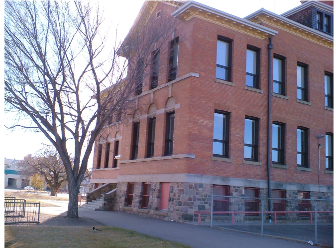
1908 building has brick masonry and stone masonry exterior walls.
