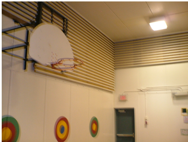
Acoustic wall panels in gymnasium.
