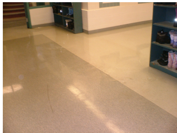
The vinyl sheet flooring in the basement corridor has uplifted with a lot of bubbles.
