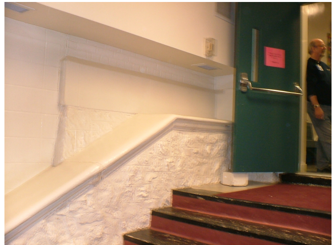
The stair with stone facing wall finish in the vestibule of the 1971 addition. This stair was constructed in 1908 for an exterior stair of the 1908 building.
