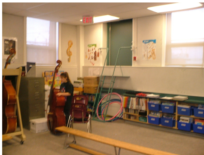
A steel framed ships ladder type stair to an exit door in a basement classroom.
