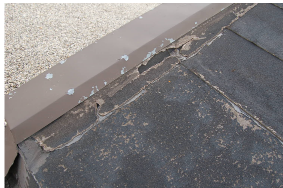
Torn and deteriorated membrane on the roof of clearstory well structure.
