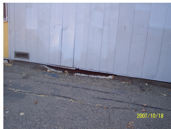
Skirting, metal siding areas damaged.
