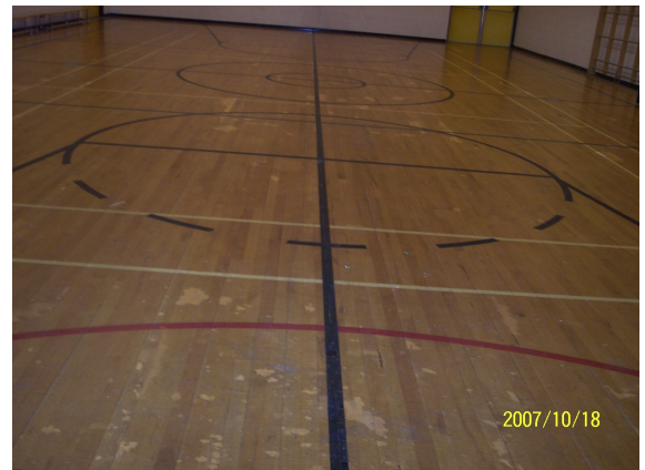
Gymnasium 13, 22 - original wood flooring has worn out.
