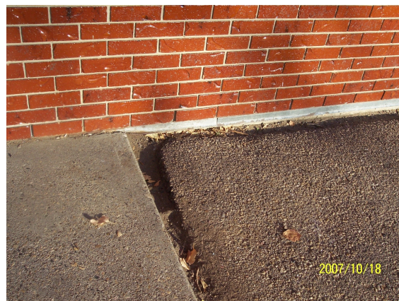
East side of building - has open gap between concrete sidewalk and paved asphalt.
