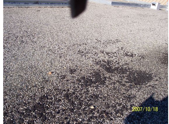
Lower roof has blisters along South corner.
