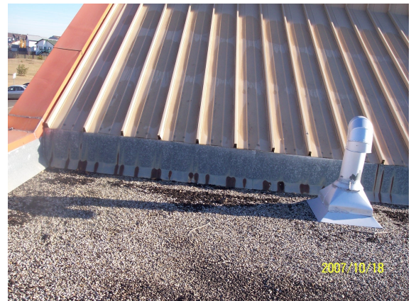
Sheet metal roof - does not have closures and has rusty flashing base.
