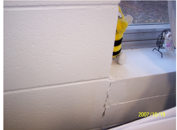
Mortar joints at window sills crack.
