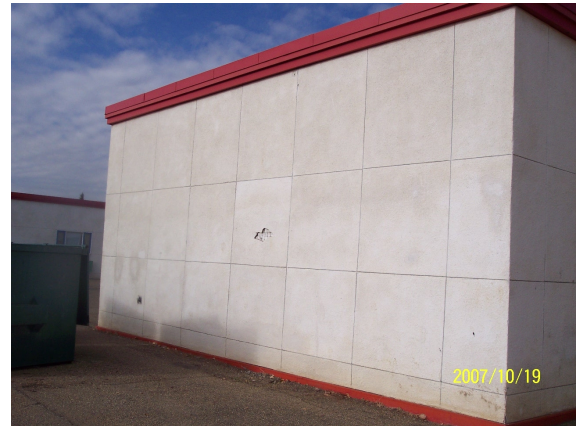
(1955) South wall of Home Economics 18 - has damaged stucco.
