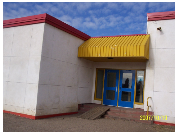
(1955) South Entrance - a wood ramp is steep and does not have proper handrails.
