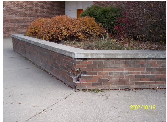
Brick planters are damaged.
