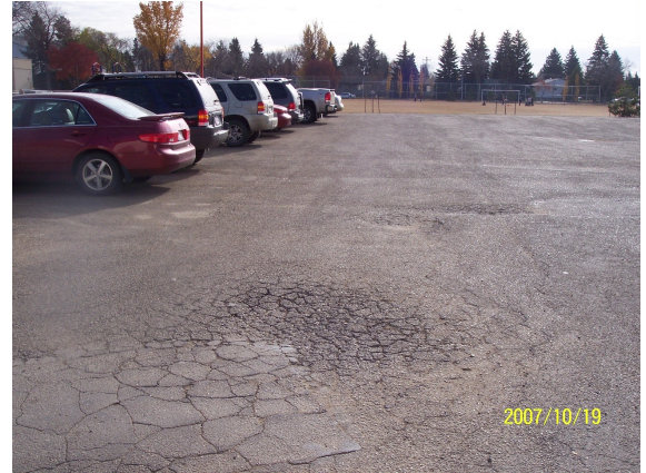
Parking lot has damaged asphalt paved spots.
