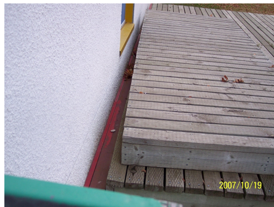
(1955) Classroom 50 has damaged wood deck.
