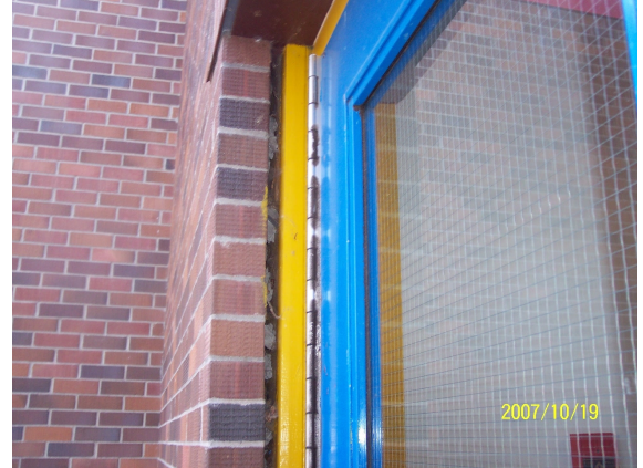
(1955) North Entrance door jamb separated from brick wall.
