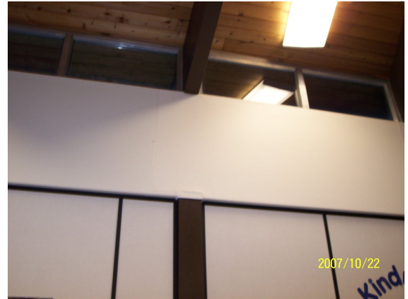
Library - sloped roof - has 64 mm T & G wood deck on glulam beams and glulam columns.
