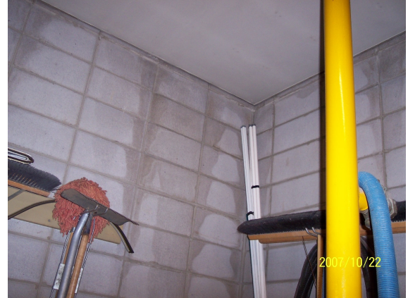
Mechanical Room 39 - has water marks on exterior concrete block walls.
