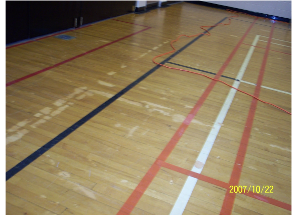
Gymnasium 39 - original wood flooring is worn out.
