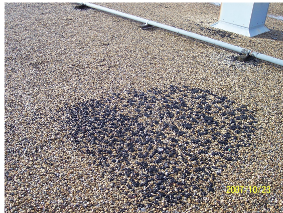
Built-up roofing has blisters.
