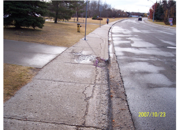
Concrete curb cut was not suitable for barrier free access.
