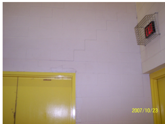
GYM 128 - mortar joints crack.
