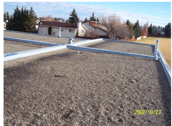
Built-up roofing has blisters.
