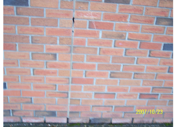
Facing brick - expansion joint caulking is missing
