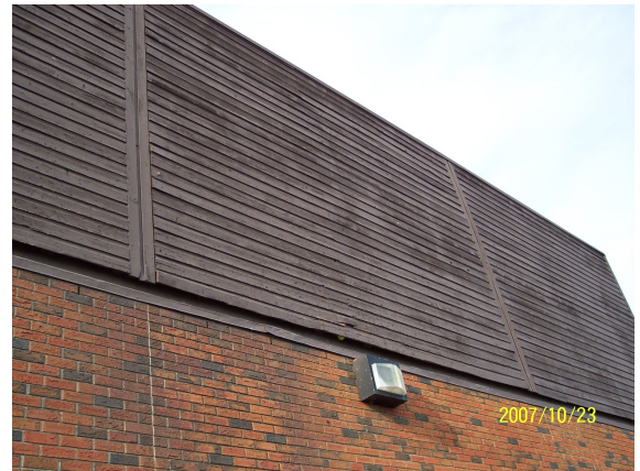
Mezzanine Mechanical Room has worn out wood siding.
