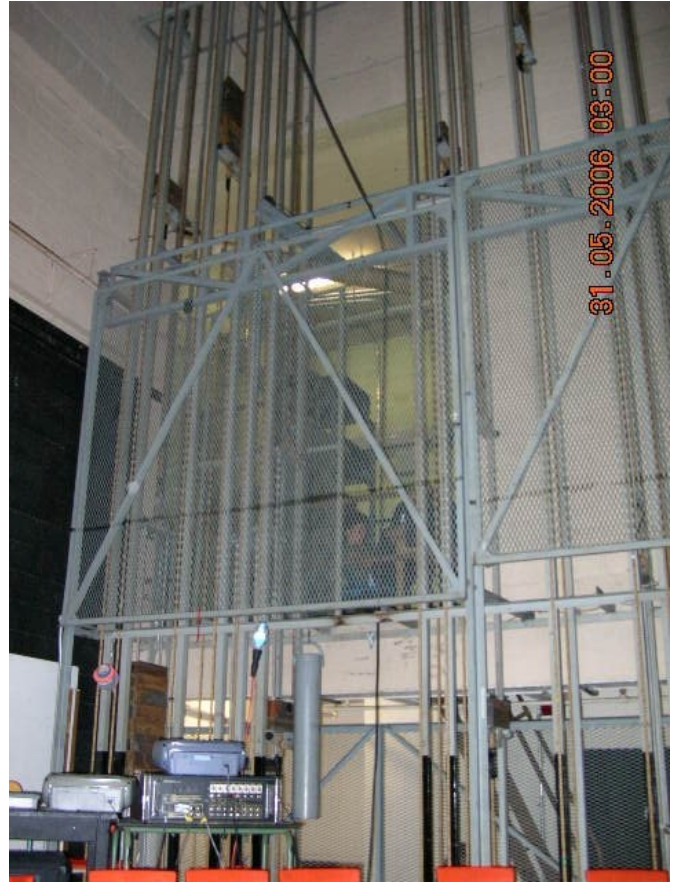
Stage counter weight and rigging system.
