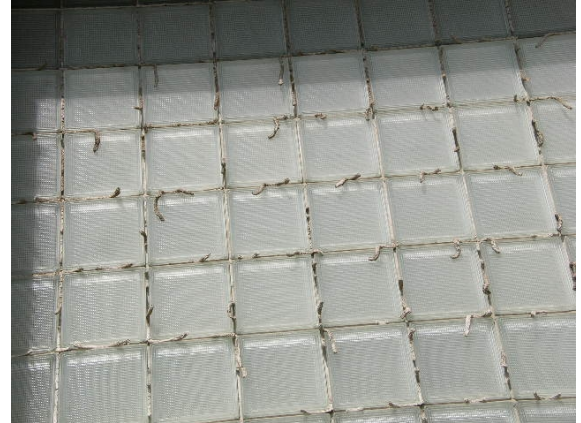
Deteriorated caulking.
