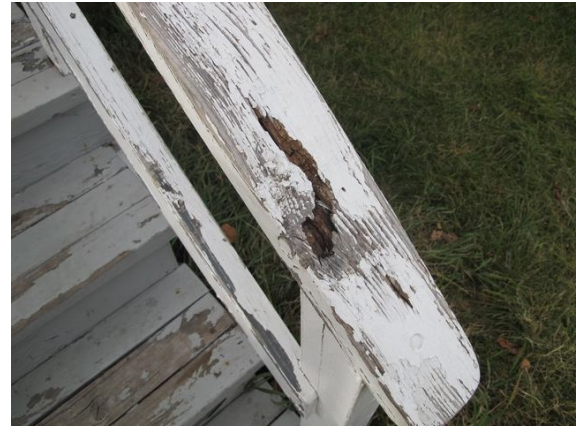
Exterior stair handrails - Portable 238
