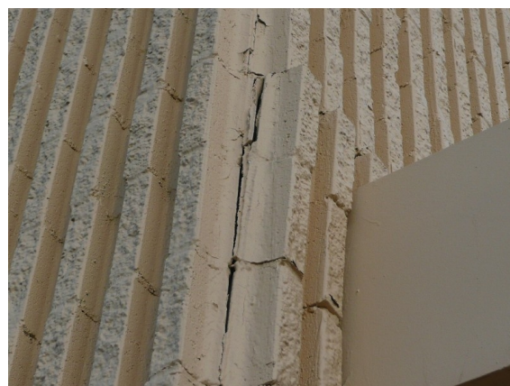
Spalling of concrete block where steel framing of canopy is bearing.
