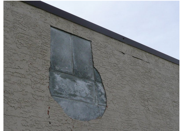
Stucco that has fallen off wall since repainting in 2009.
