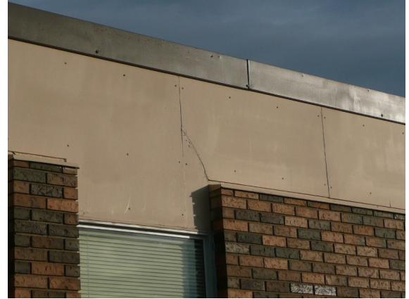
Cracks in asbestos cement panels.
