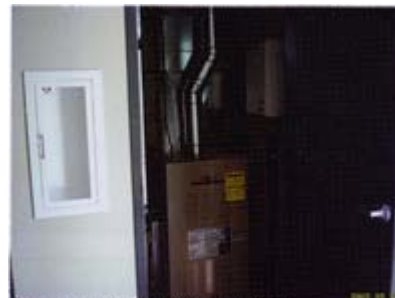
Fire Extinguisher Cabinet and Mechanical Room.
