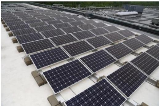
Roof mounted tilted PV array using ballasts <sup>11</sup>
