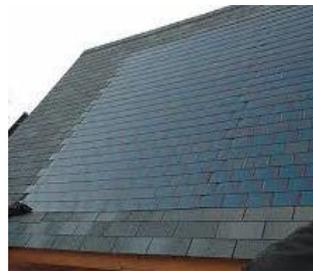
*BIPV Roof Shingles<sup>7</sup>*
