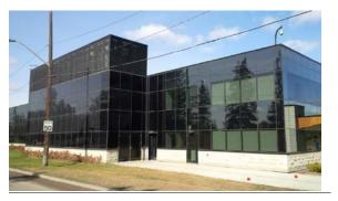
Figure 8 – Integrated PV – UofA Isotope Centre - Photo credit – V. Solbak
