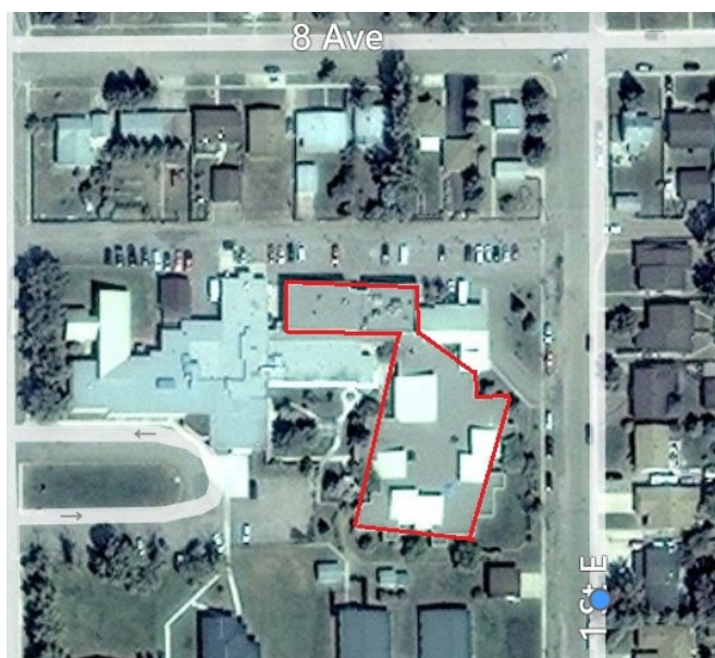
Aerial view of the Site from Google Earth. The Site assessed is outlined in red.
