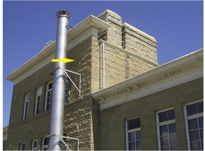
South facade. Arrow points to stabilizer anchors at penthouse floor.
