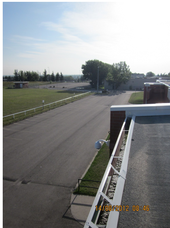
View of NE portion of rear parking and site
