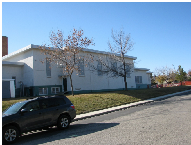
School front (north)
