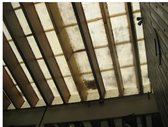
Interior view on enclosed courtyard.
