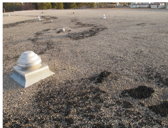
Original roof above the 1969 Addition
