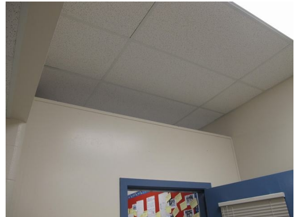
Openings between the corridor and classrooms 11 and 15.
