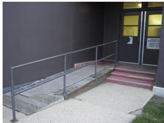
(1956) Addition (East Corridor Entrance) - wood ramp is rotten and handrail is not up to barrier free standards.
