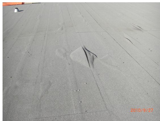
(1956) Addition (Classrooms) - SBS roofing has bubbles. (approx. 500 sq. m.)
