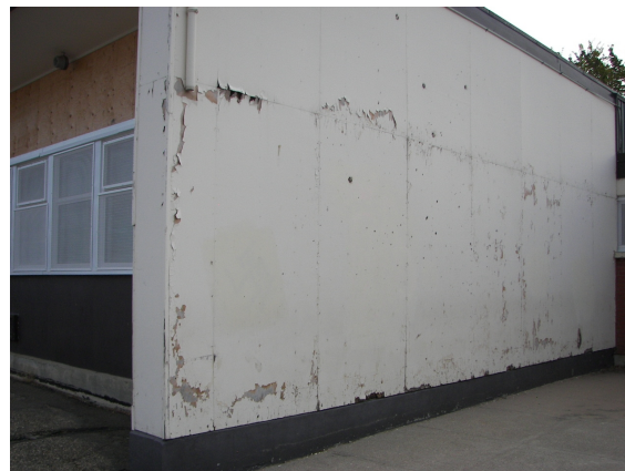
(1955) Original Building (South End Wall) - has damaged plywood finish.
