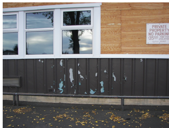
(1955) Original Building (North Lower Wall of Library 93; East Lower Wall of Classrooms) - have damaged vertical corrugated asbestos panels.
