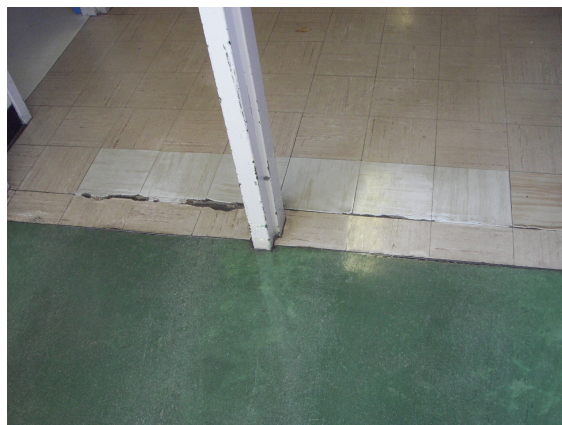
(1961) Addition (Corridor connecting to 1955 section) - has cracked floor slab.
