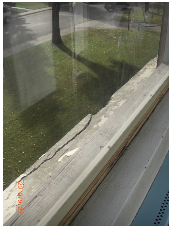
(1961) Addition (Upper Floor - Classroom 40)- wood windows have worn out.
