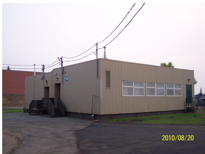
(1991) Portable (238) - Southwest Elevation.
