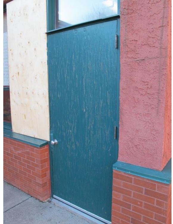
Deteriorated wood door assembly.
