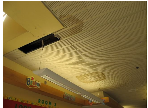
Missing and stained ceiling tiles in the main corridor.
