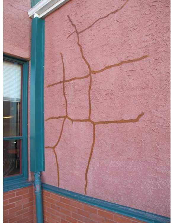
Cracks on stucc wall assembly.
