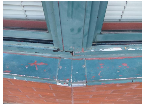
Deteriorated sealant along window assembly.
