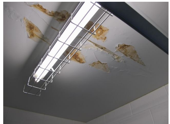
Damaged ceiling in girl's change room.
