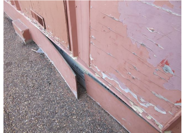
Deteriorated skirt and wood panels.
