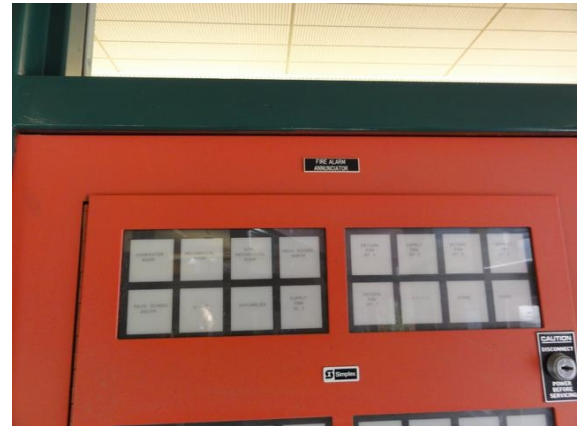
Remote fire alarm annunciator at main entrance.
