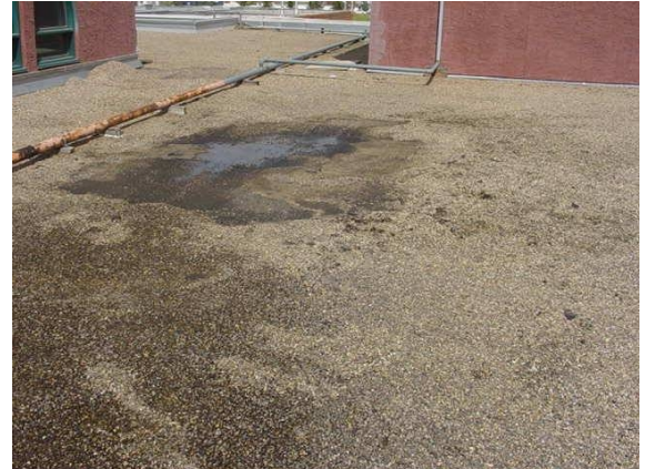
Typical condition of Built-up roof assembly.
