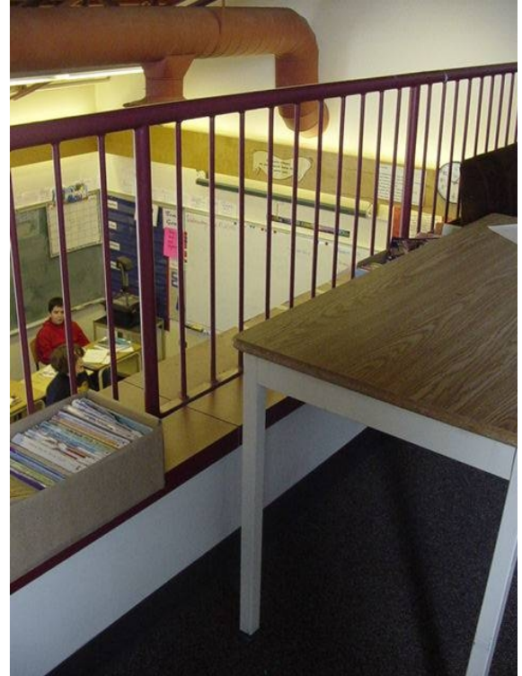
Railing height on mezzanine does not meet building code.
