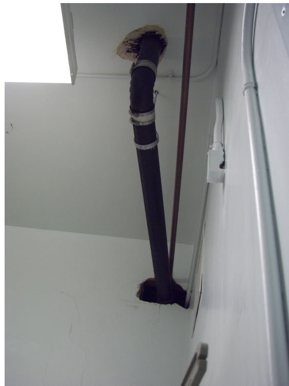
(1946) Original Building (Main Floor - Storage 26) - has space around pipe penetration.
