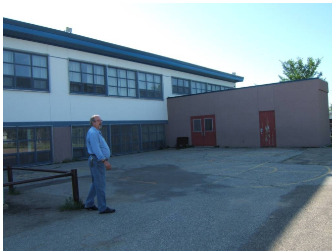
West elevation of school and storage facility.
