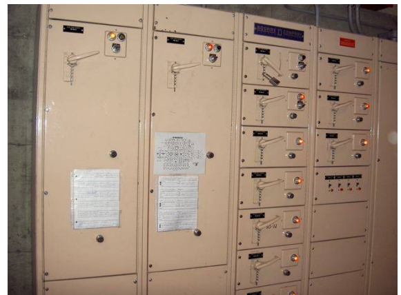
AGED SQUARE D MOTOR CONTROL CENTRE
