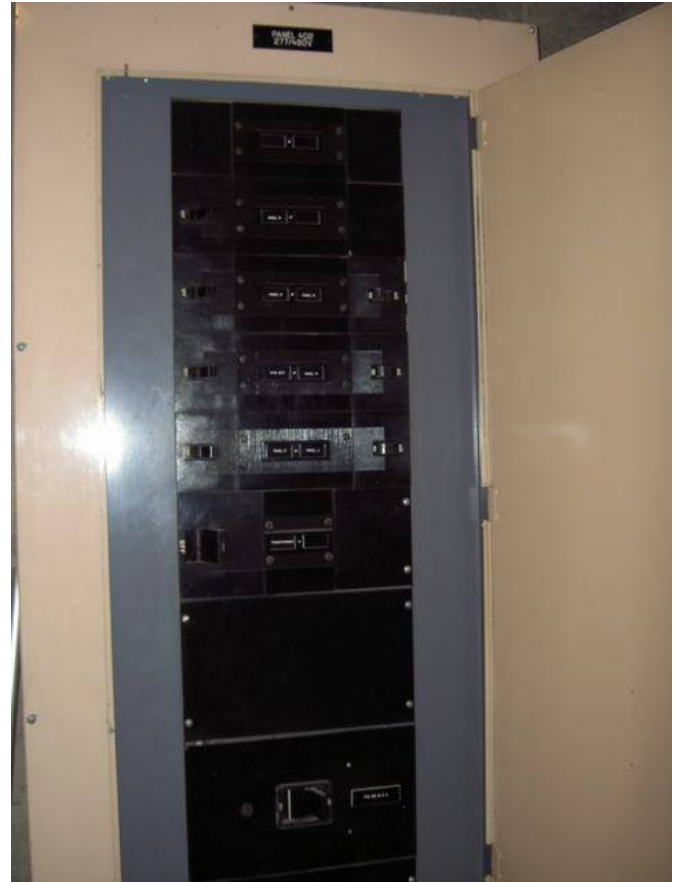
Aged distribution panel.
