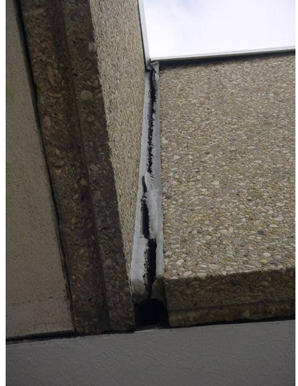
DETERIORATED SEALANT AND SHIFTING FASCIA PANELS
