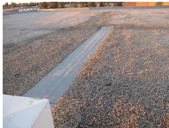
Ongoing repair on the upper roof areas.
