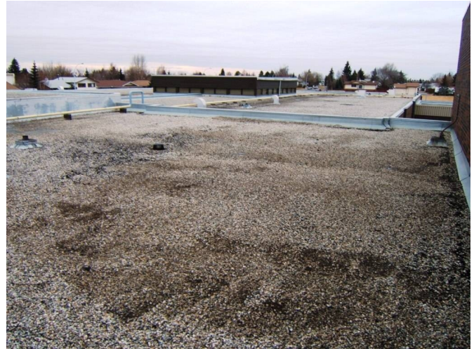
Partial view of built-up roofing.
