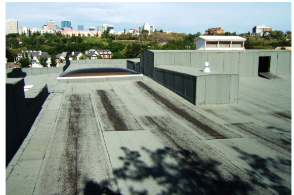
View of SBS roof.
