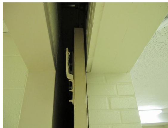
Pocket fire rated doors between the 1956 & 1966 Sections
