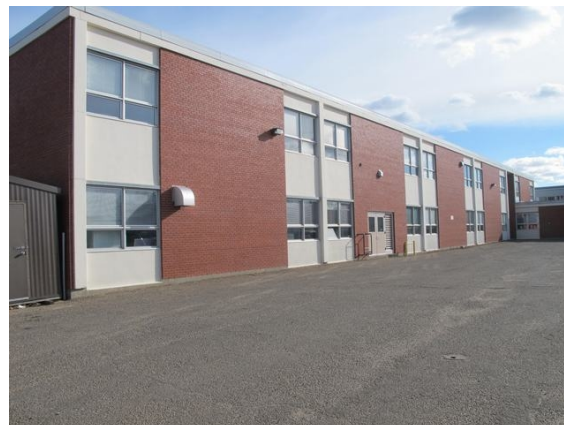
Original windows in 1966 Section.
