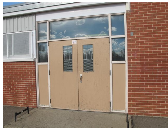
Typical condition of wood framed entrance doors & assembly.
