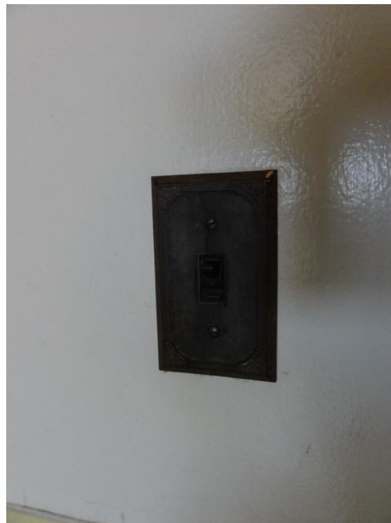
Aged light switch with bakelite coverplate.
