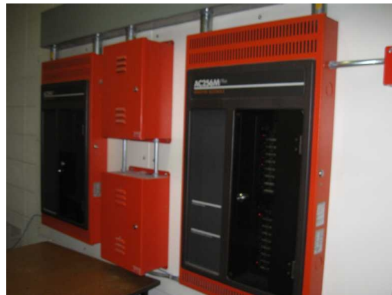
Andover model AC256 main control panel
