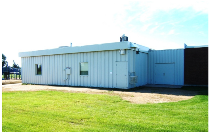
North Elevation of 1974 and 2003 Portable Units
